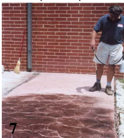
7/ Application des Acid Stains
